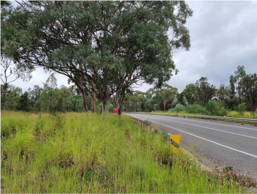
Plate 2.7 Overgrown vegetation and street trees restricting sight distance on Thomas Mitchell Drive
