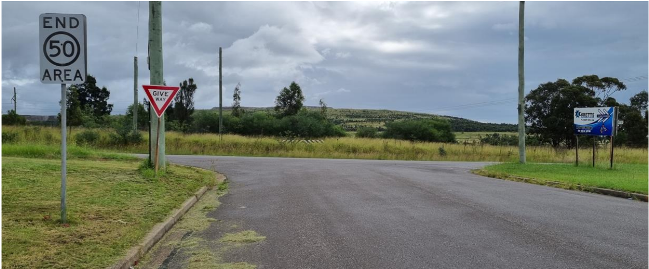
Plate 2.9 No 'Giveaway' line marking
