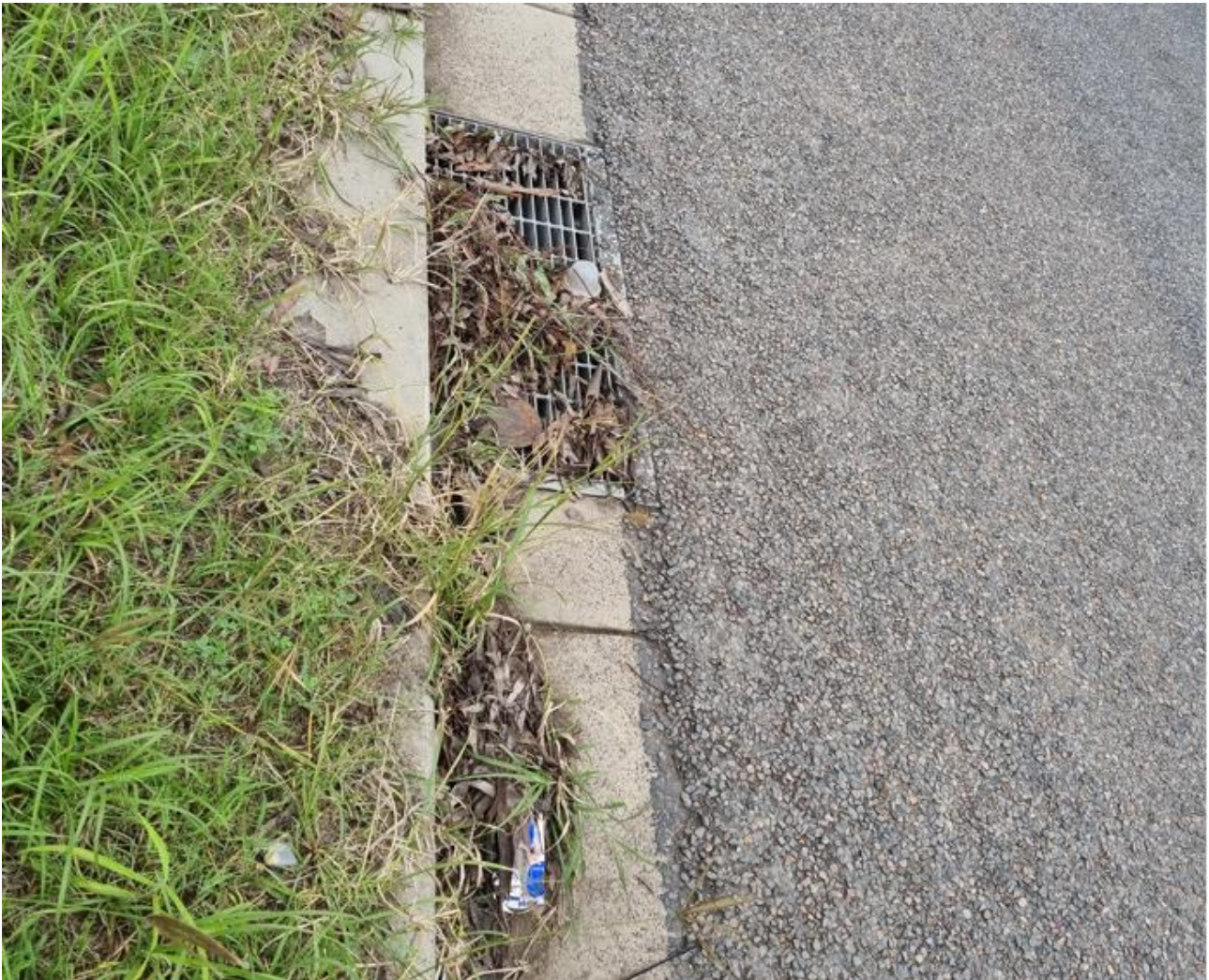
Plate 2.5 Uncleaned drainage pit located on eastern side of Thomas Mitchell Drive, south of Glen Munro Road
