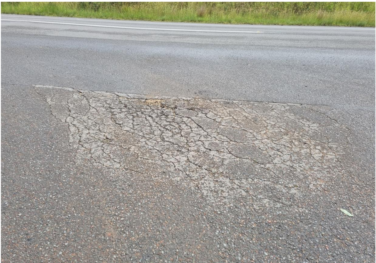
Plate 2.4 Cracked pavement on the southern side of Glen Munro Road at Thomas Mitchell Drive intersection
